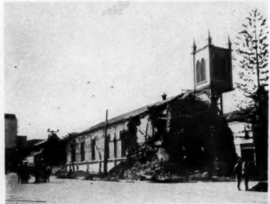
FIG. 11. CATHOLIC CHURCH, SHOWING DESTRUCTION OF ADOBE BUILDING, BRICK VENEERED
